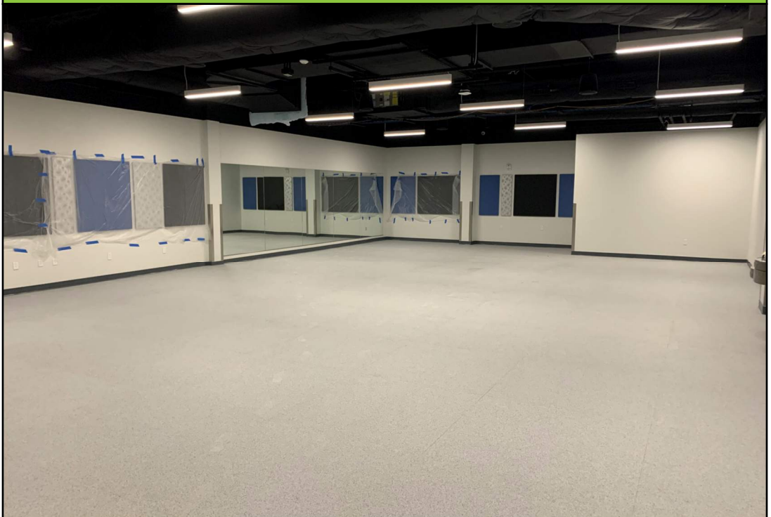
Completed laying Athletic Resilient Flooring in Levels 1 & 2
