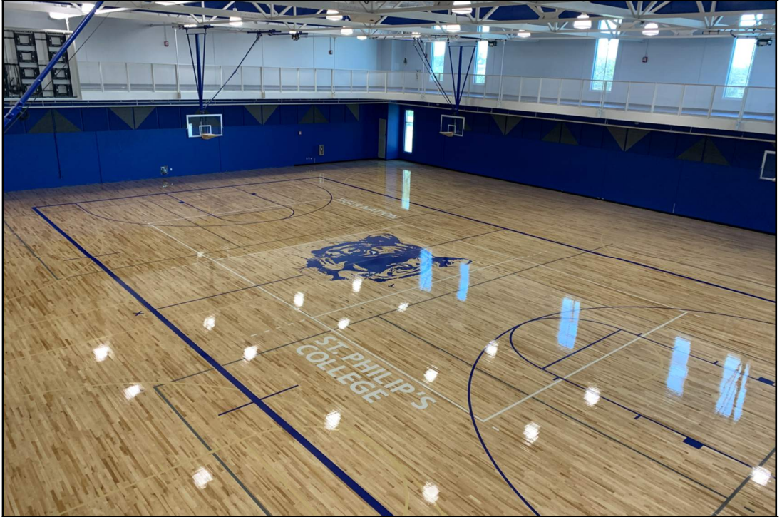
Completed laying Athletic Resilient Flooring in Levels 1 & 2
