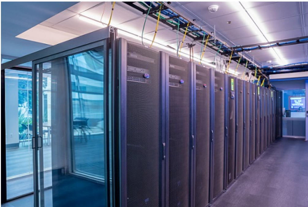
Figure 11: Web Services Classroom
