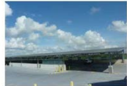
Northwest Vista College – Parking Garage
